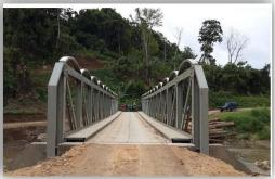
Hornibrook NGI was contracted by New Ireland Provincial Government to fabricate and supply our Standard Two (2) 36m Panel Bridge. We provide technical support to the local civil contractor to during construction.
